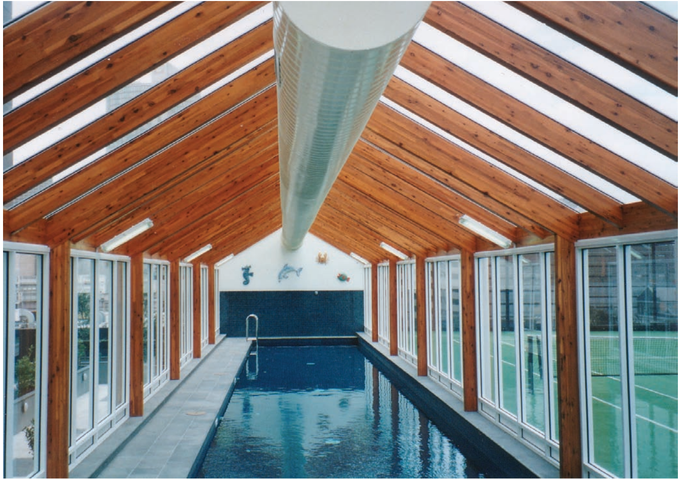
■ Central Equity GL10 DuraBeam portals, Southbank.
